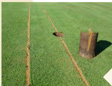
This cross section shows how the groove is filled with sand up to 15-20cms deep.
